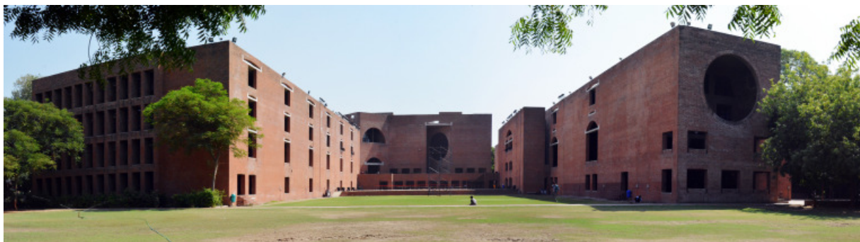
Fig. 24: The Louis I Kahn Plaza, as seen from the northwest. The Library is seen in centre, with the Classroom Block on the right and the Faculty Wing on the left
