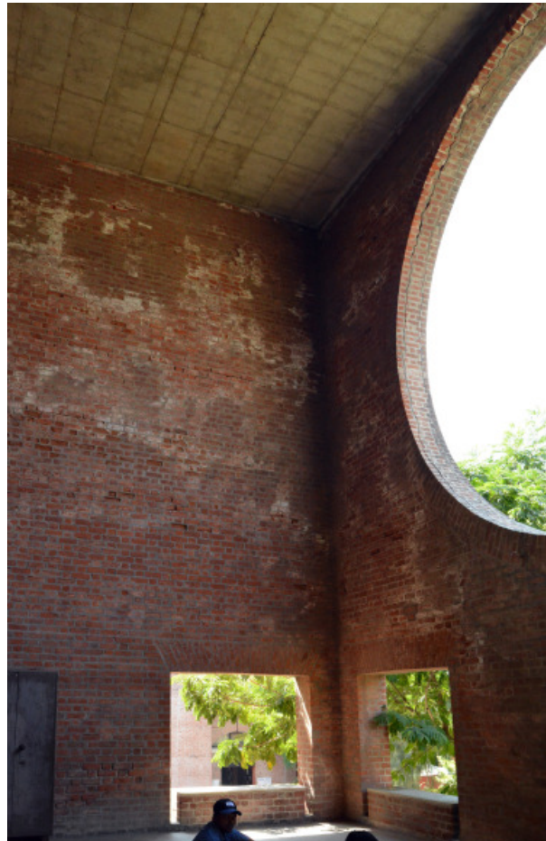
Fig. 16, 17, 18, 19: Instances of deterioration caused by defects of the original materials and construction, patch repair methods, and lack of routine maintenance. One can see damage due to rising damp, seepage of water through damaged roof terracing, and rusting of steel bars embedded in brickwork.
