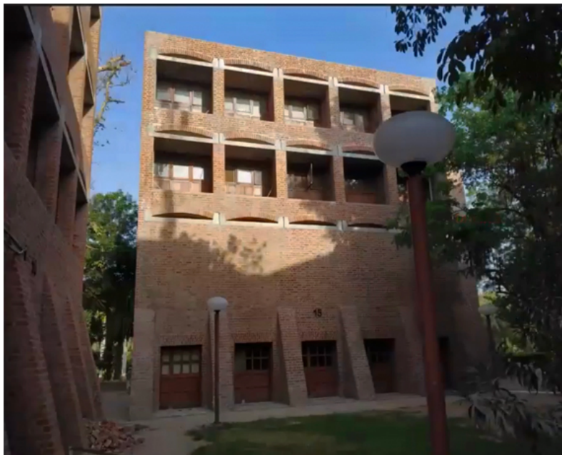
The completed civic and structural restoration of dormitory D-15
