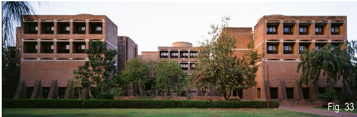
Fig. 31, 32, 33 (Above): The cluster of Dormitories for 'Unmarried Students'. Bearing walls splayed out at lower levels to become buttresses to withstand outward thrust of large span arches. Reinforced concrete ties used for segmental arches became a significant attribute of IIM-A's architectural vocabulary and aesthetic appeal.
