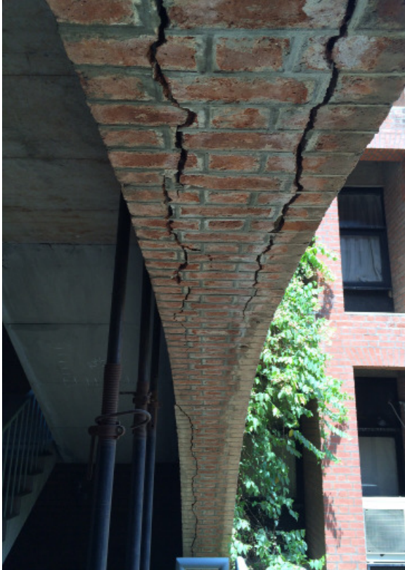
Fig. 16, 17, 18, 19: Instances of deterioration caused by defects of the original materials and construction, patch repair methods, and lack of routine maintenance. One can see damage due to rising damp, seepage of water through damaged roof terracing, and rusting of steel bars embedded in brickwork.
