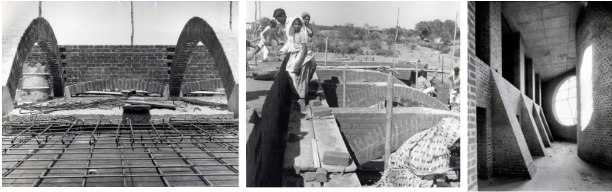
Figs. 43, 44, 45 Archival images of construction showing various types of arches and buttressed supports.
