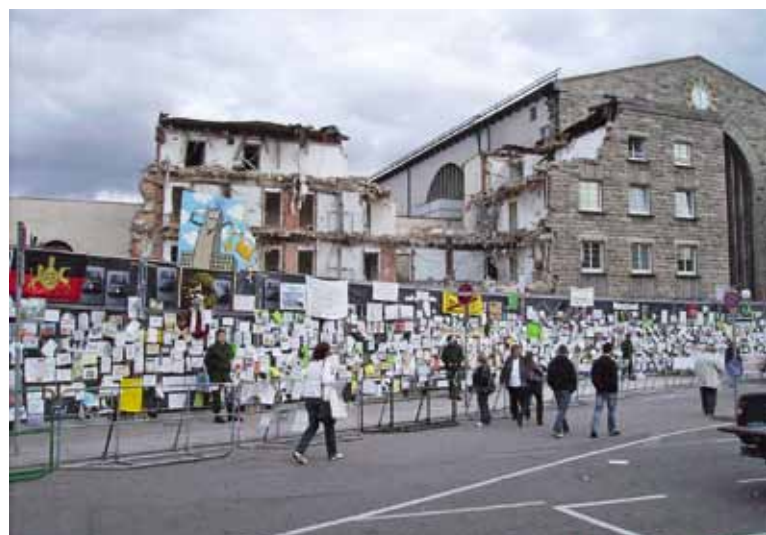
Stuttgart Central Station, demolition of the north wing (photo: V. Eidloth)
