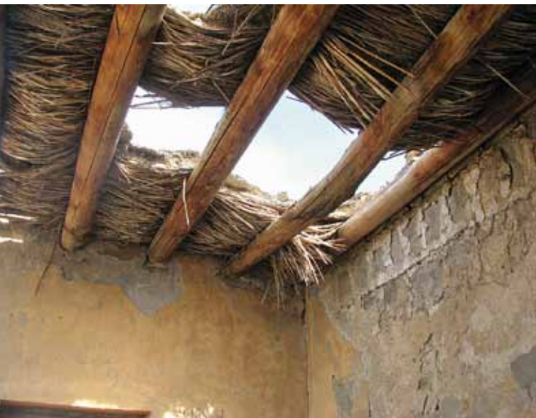
Erebouni Fortress, damaged wall paintings
