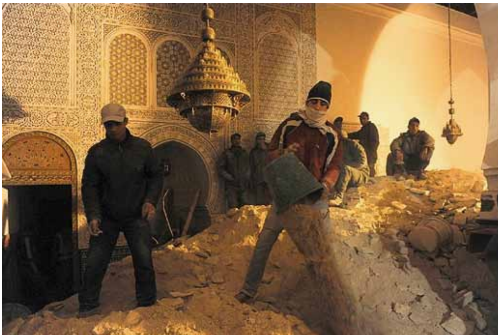
Workers removing the rubble inside the mosque
