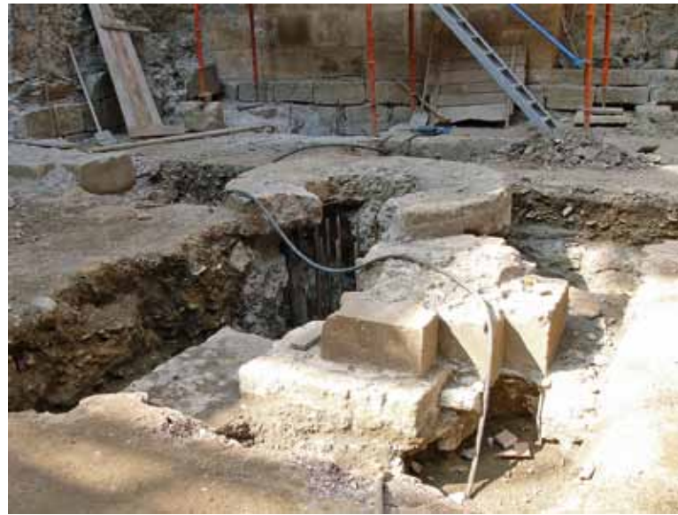
Authentic column bases perforated for the arrangement of concrete piles
