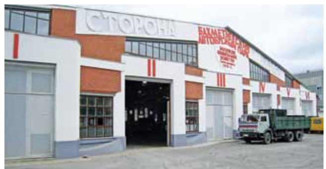
Bakhmetevsky Garage (1926–27) after reconstruction, 2009 (photo: A. Zalivako).
