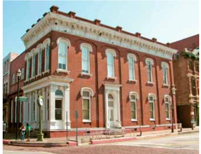
Galveston, Texas, typical late 19th century building
