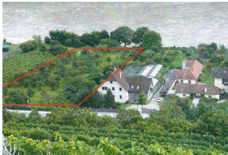
Storage halls for mobile flood protection
