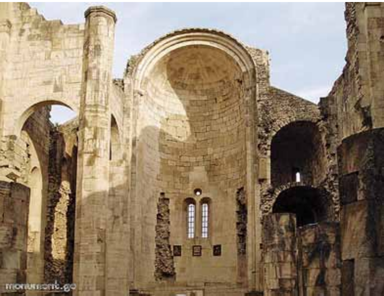
Bagrati Cathedral, the interior before intervention
