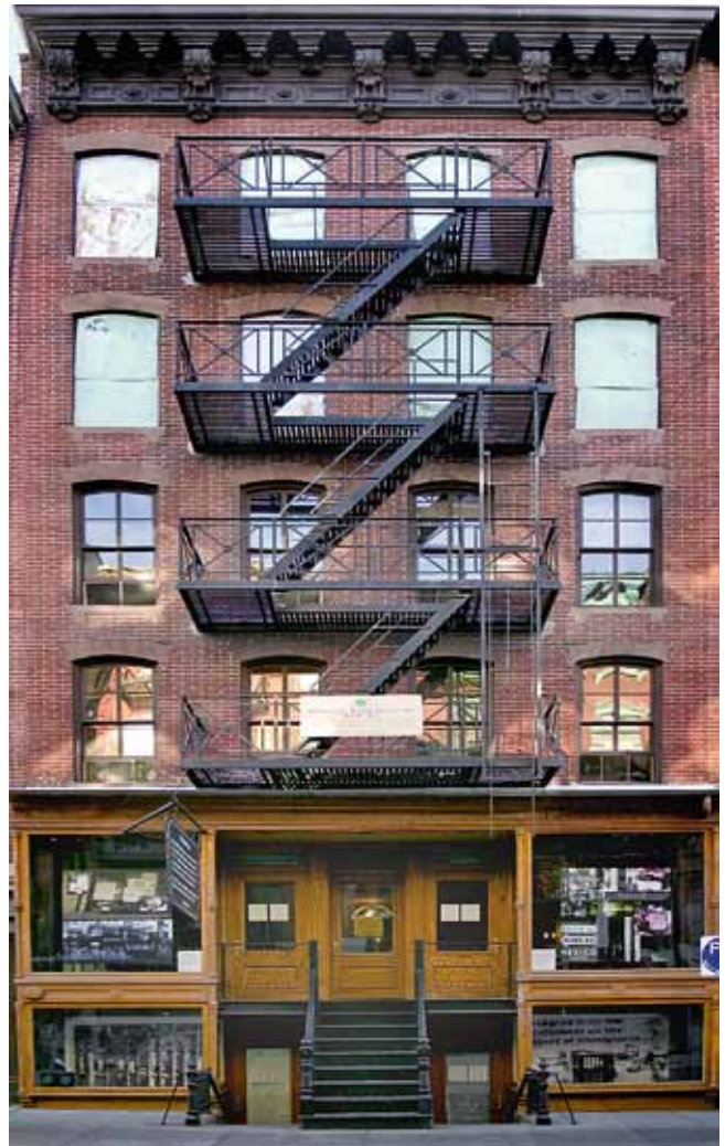
The Lower East Side, New York City, typical façade
