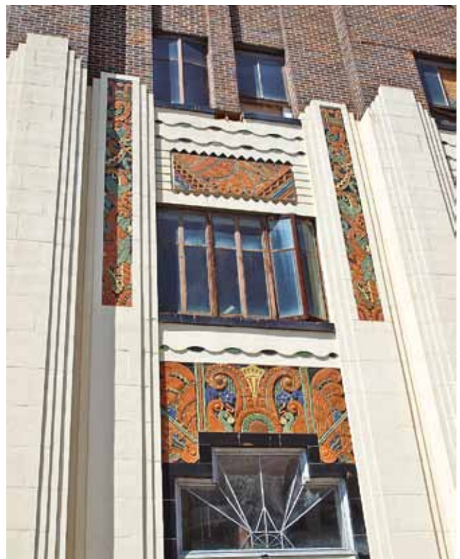
Threefoot Building, detail of the façade
