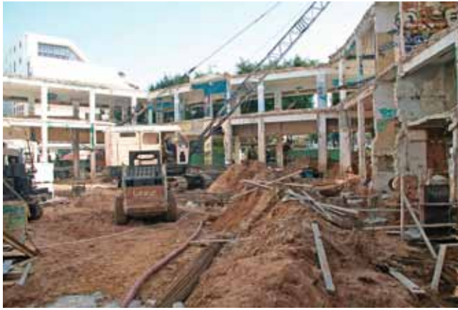
Building on Dizengoff Square, beginning of demolition work on the courtyard side (photo: B. Furrer)
