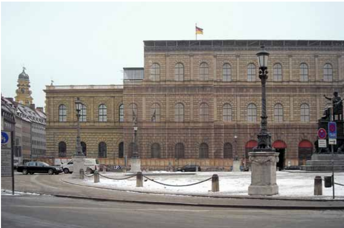
Munich, covering in front of the façade of the Residence (photo: I. Cisek)
