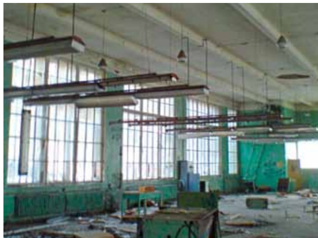
El Lissitzky, Zhurgaz printing house, The site in November 2010
