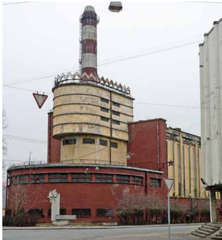
Krasnoje Znamja Textile Factory, powerstation (photo: A. Zalivako)
