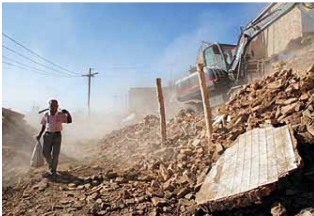
Bulldozer razing part of Old City and resulting debris (source: www.chinadigitaltimes.net)
