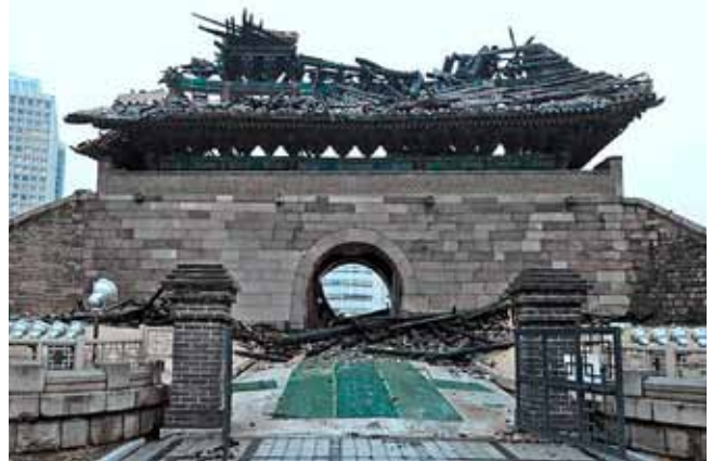
The gate immediately after the fire
