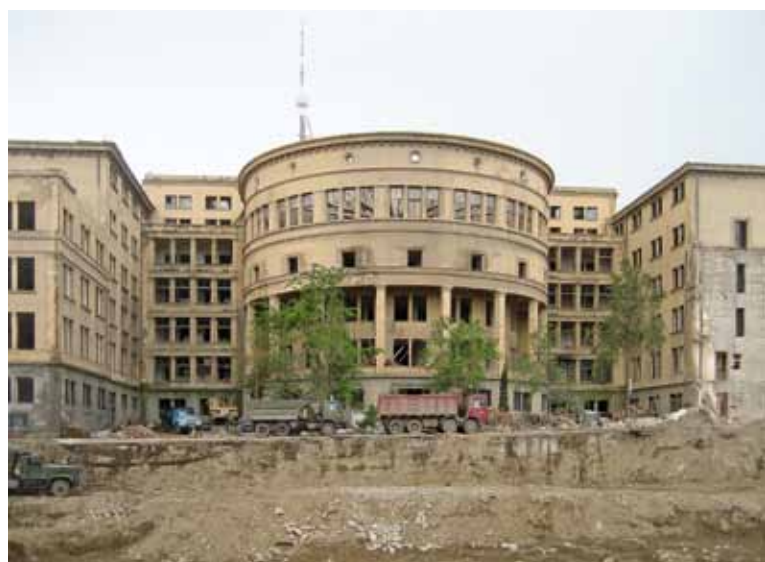
IMEL building, back façade (photo: M. Mania)
