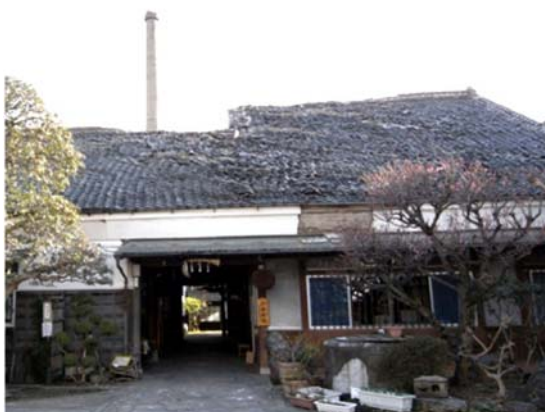
Figure 2.25 A traditional building in Makabe (Top: Before earthquake; Bottom: After earthquake)
