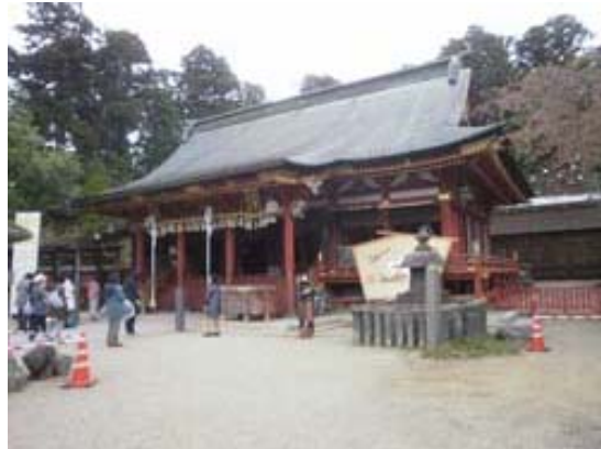
Figure 2.17 The Shiogama Shrine, an important cultural property: Undamaged
