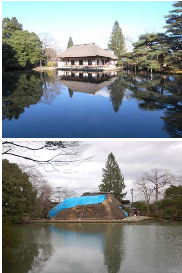
Figure 2.39 Yubikan (Top: Before earthquake; Bottom: After earthquake)
