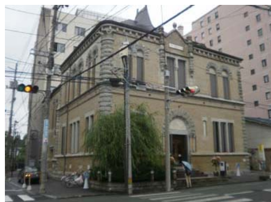
Figure 2.19 Former 99 Bank Head Office, an important cultural property: Minor damage to internal walls and ceiling
