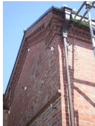
Figure 2.21 Disaster-affected brick storehouse, the Machikado Kura Nomura (Top: Building exterior; Bottom: Cracked gable wall)
