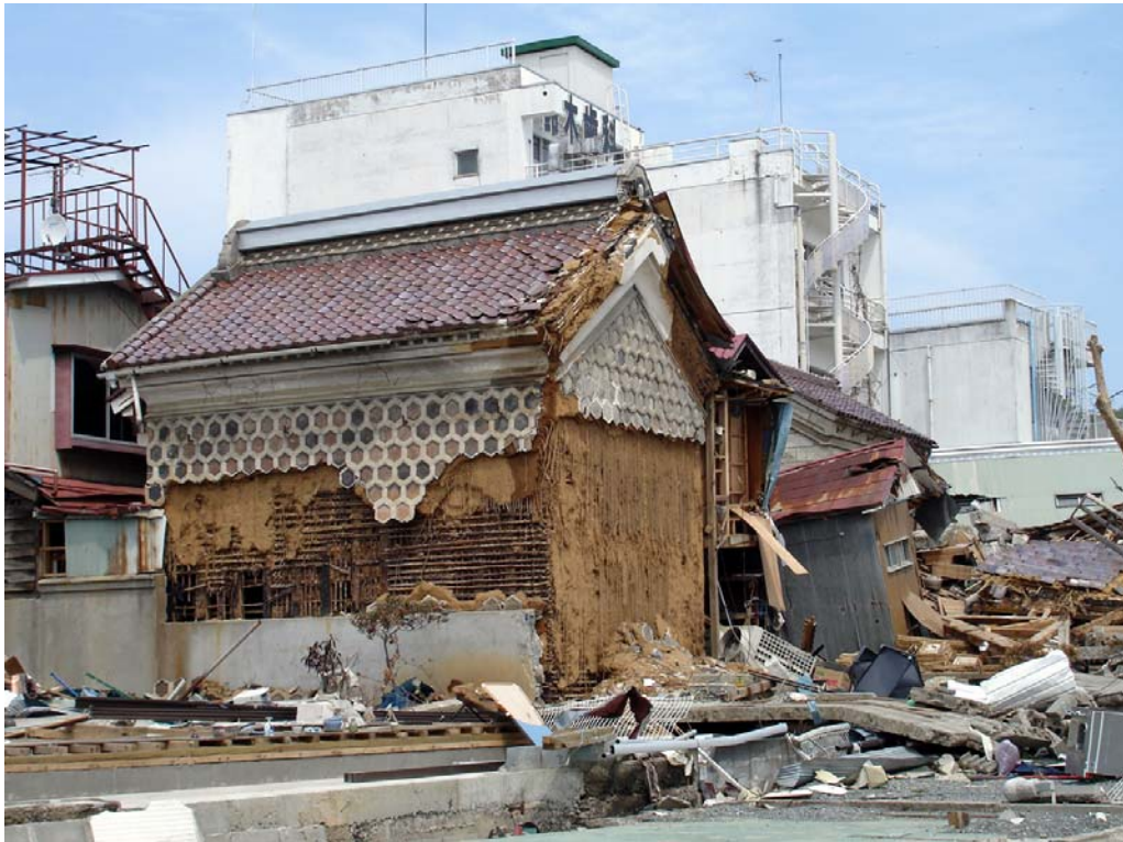
Collapsed buildings (Kesennuma City, Miyagi Prefecture )
