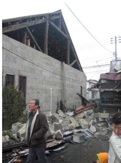
Figure 4.4 External appearance of the Sekinoichi Brewery's earthen warehouse ( Torigura )
