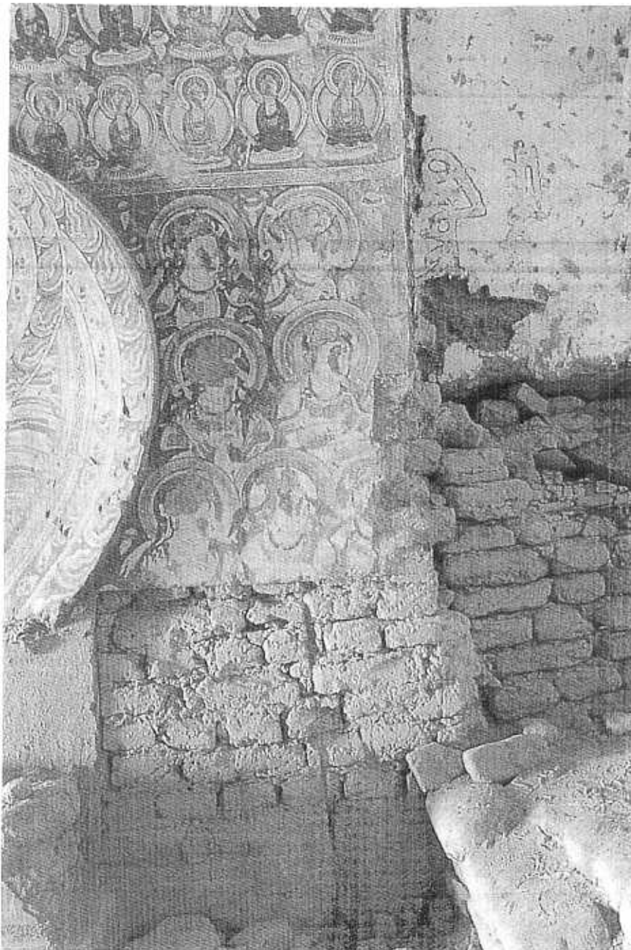
Painted gypsum panels and sculpture on a mud-brick background. (De Gao, China).
