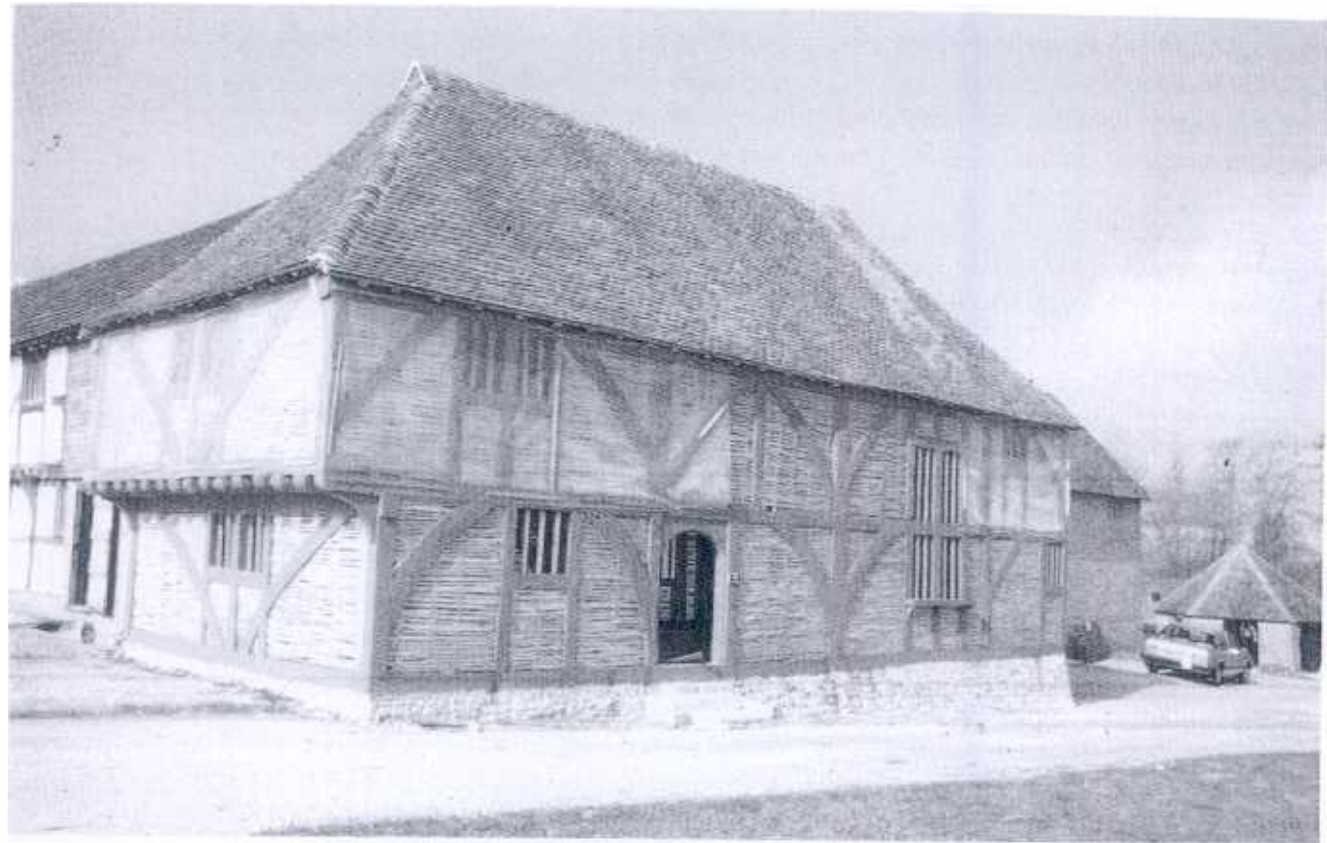
Wattle panels in timber framing awaiting application of daub. (Chichester, England).
